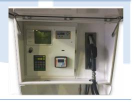
The card reader is placed in the middle of the control panel. When a chip card is placed close to the card reader and the system will be authorized to deliver fuel.
