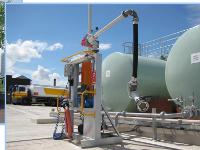
...700 Series meter in a loading rack
